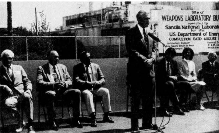
APRIL 10, 1985, saw Sandia break ground for the long-awaited Weapons Engineering Laboratory, a 77,000-square-foot, three-story building due for occupancy by the fall of 1987. Former DOE Assistant Secretary for Defense Programs Major Gen. William Hoover addressed Sandians gathered for the ceremony just south of Bldg. 911. Seated on the platform were (from left) Dick Claassen (8000), LLNL Director Roger Batzel, DOE San Francisco Operations Office Manager Dick DuVal, Livermore Mayor Dale Turner, Livermore Chamber of Commerce President Sue Dell'Acqua, and Garland Bryan of Flatow, Moore & Bryan architectural firm.
